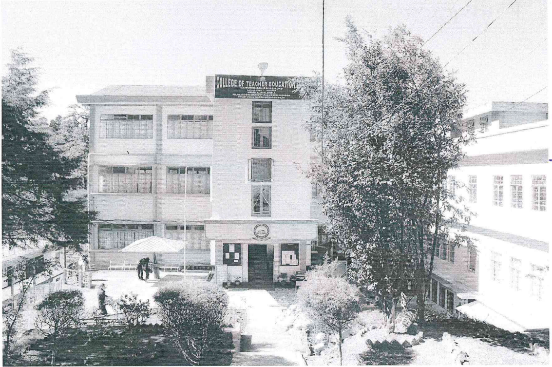
Front view of the Building
