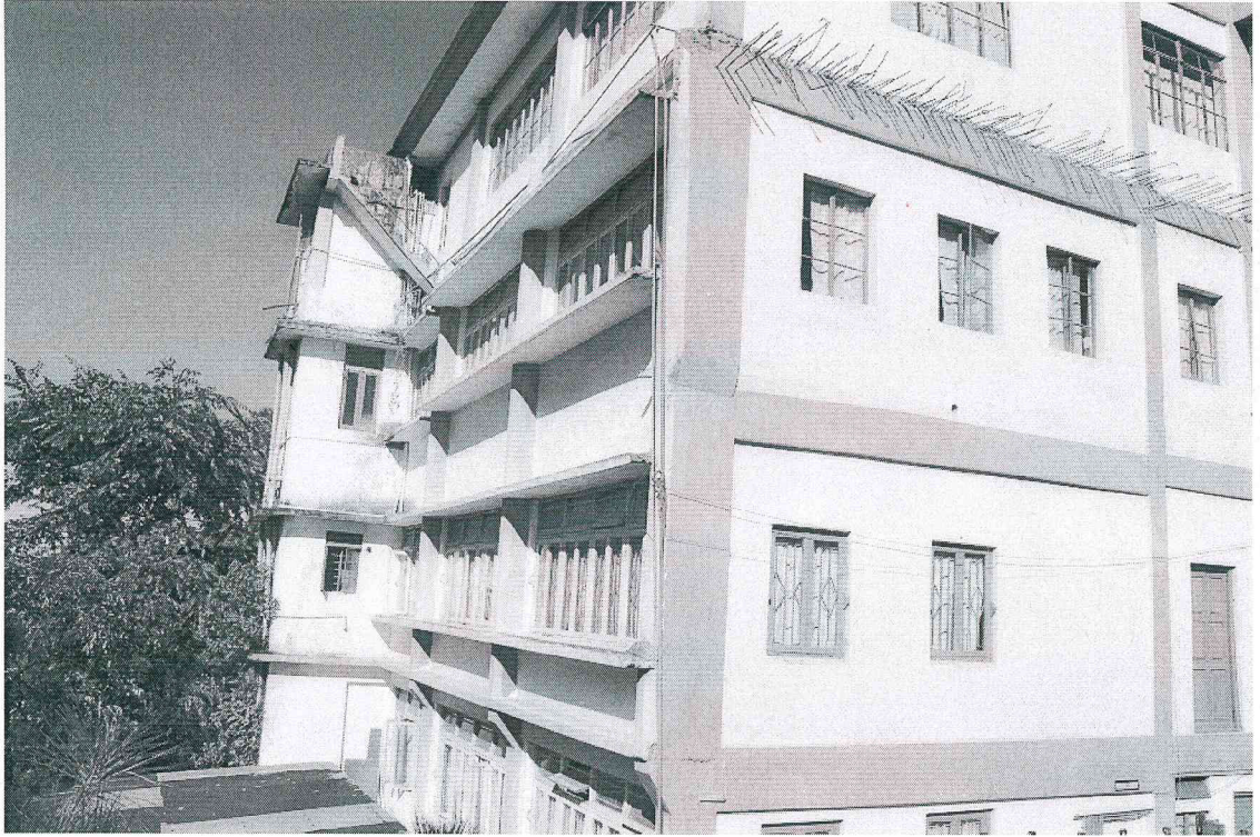
Rear view of the building
